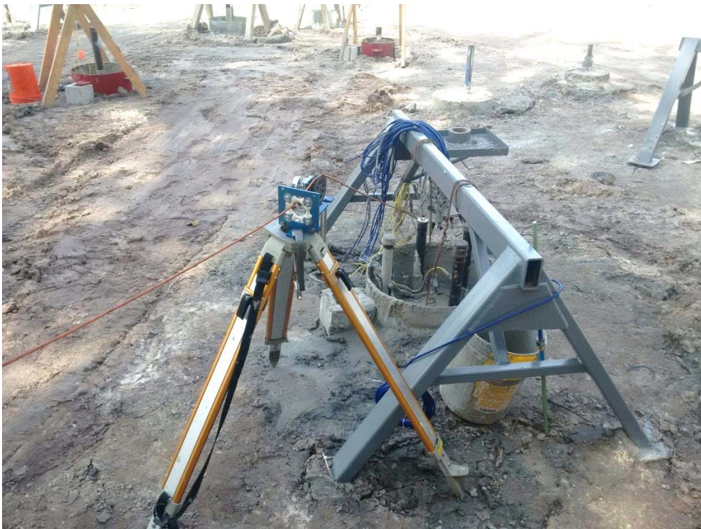
Figure 2.11 Probe testing pile C2 at approximately 24hrs after pile installation.
