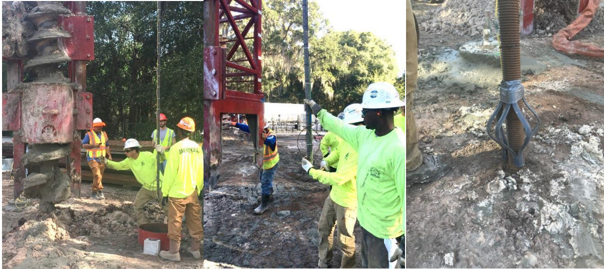
Figure 4.4 Number 8 bar with weak and widely spaced centralizers over 10ft (left).
