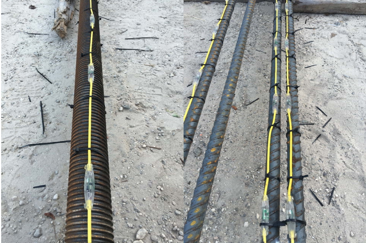
Figure 2.8 3in center bars (left) and #11 center bars (right) instrumented with thermal wires.
