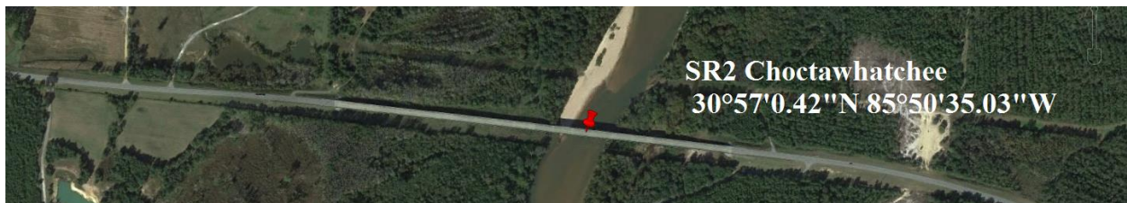
Figure 4.11 Bridge Number 520145 (SR2 Choctawhatchee Bridge) plan image.
