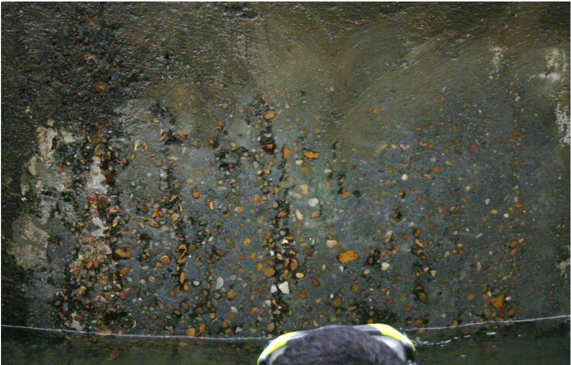
Figure 4.59 East side of test shaft 8 post-cleaning.
