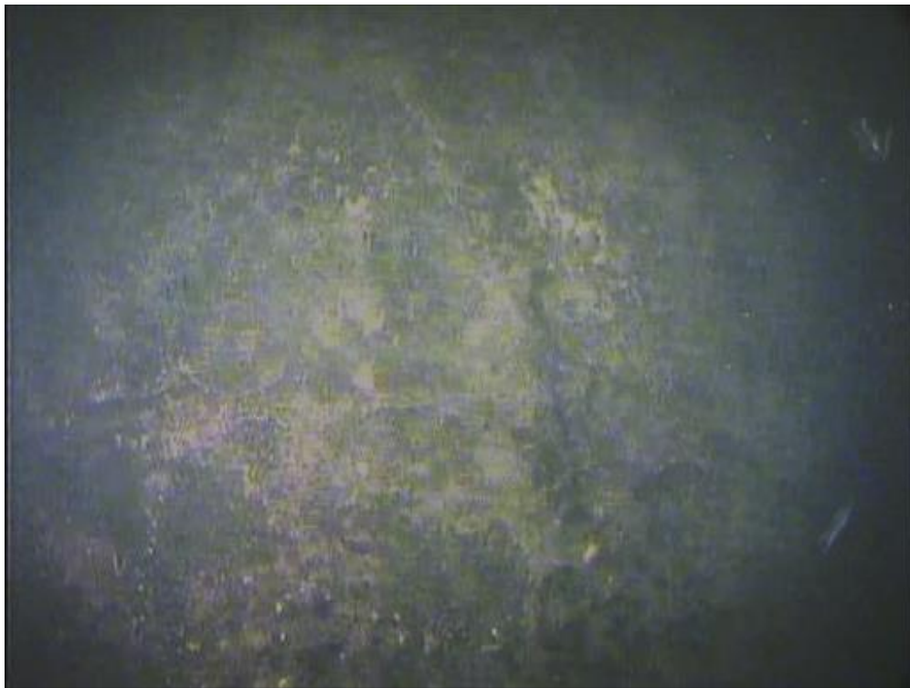
Figure 4.54 Shaft 58-1 prior to cleaning
