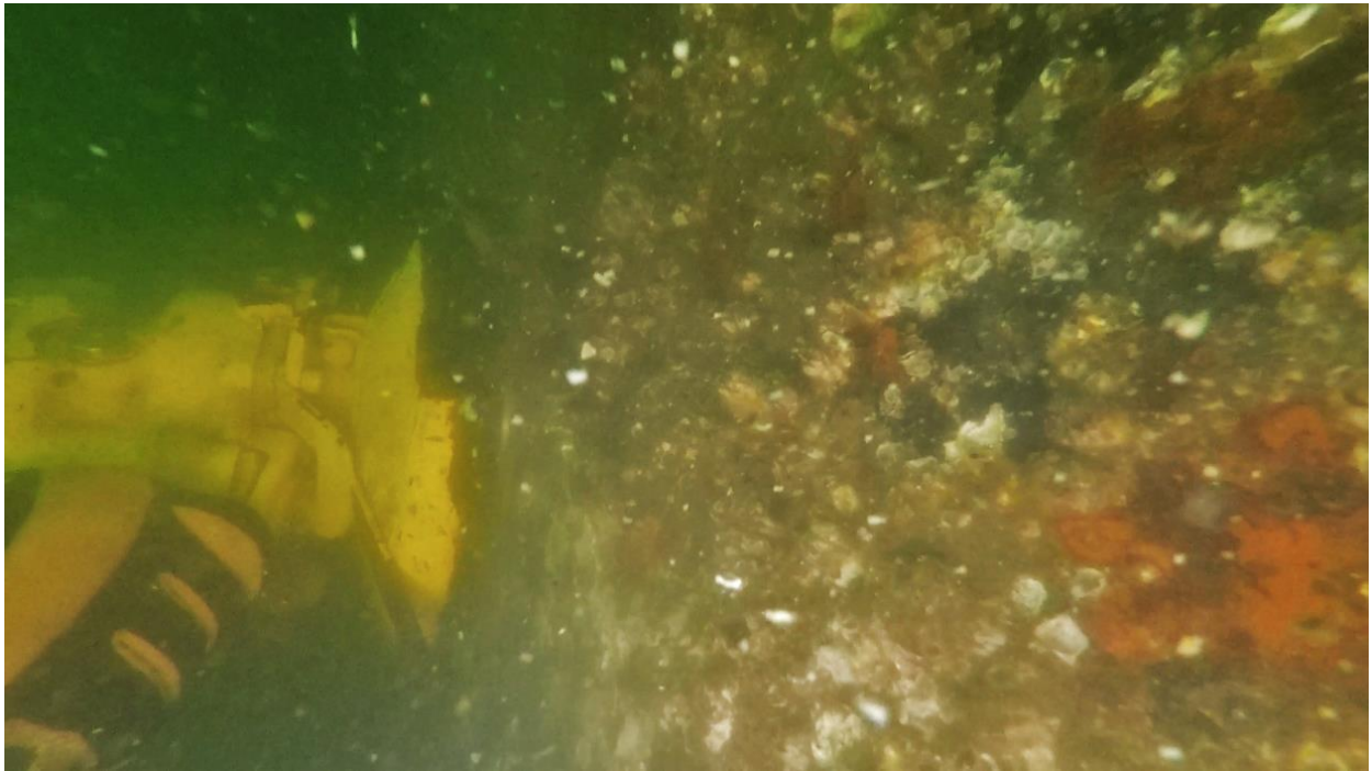
Figure 4.28 Shaft 94-4 during cleaning with the grinder
