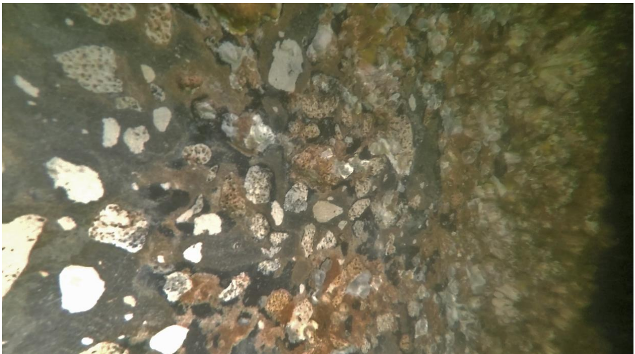
Figure 4.34 Shaft 84-4 partially cleaned, note clean concrete going into layer of barnacles
