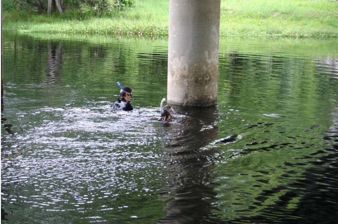
Figure 4.46 Diver follow-up to further review column-to-shaft interface.
