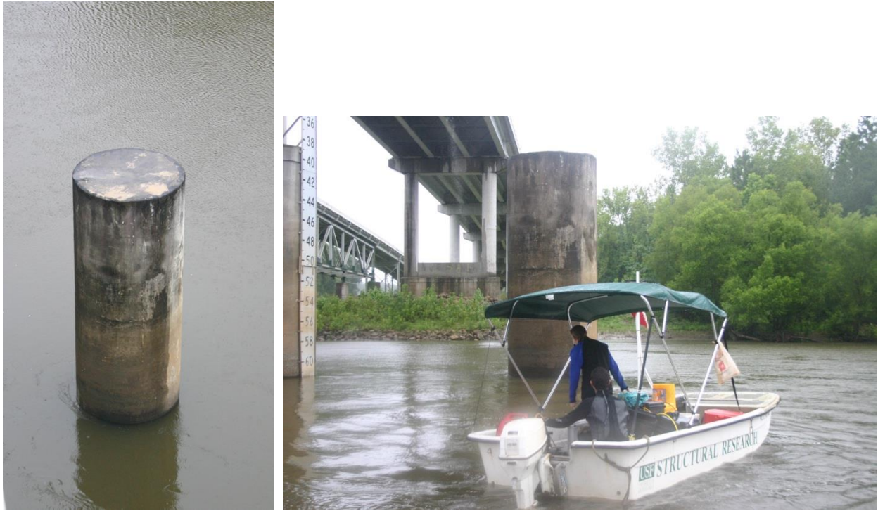
Figure 4.56 Test Pile adjacent (west) of Pier 59
