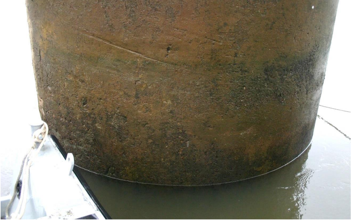
Figure 4.58 East side of test shaft 8 pre-cleaning.
