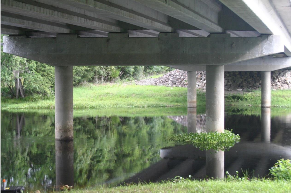
Figure 4.44 Four water column-to-shaft structures.
