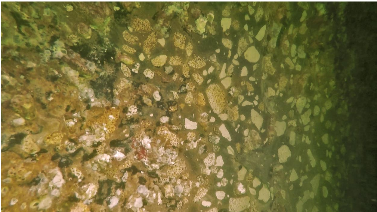
Figure 4.36. Cleaned portion of 84-4, east side of shaft
