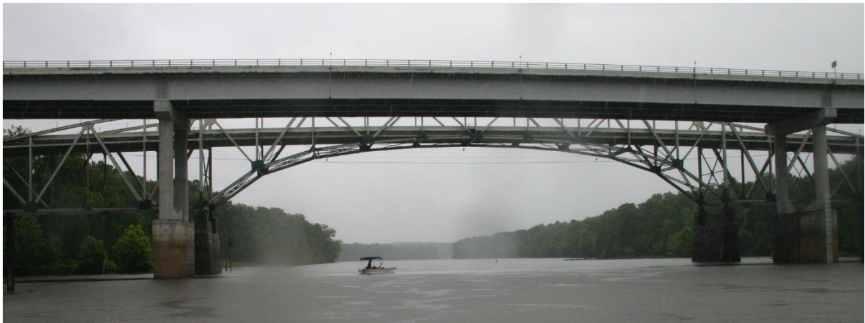
Figure 4.48 Main span of the Blountstown Bridge.
